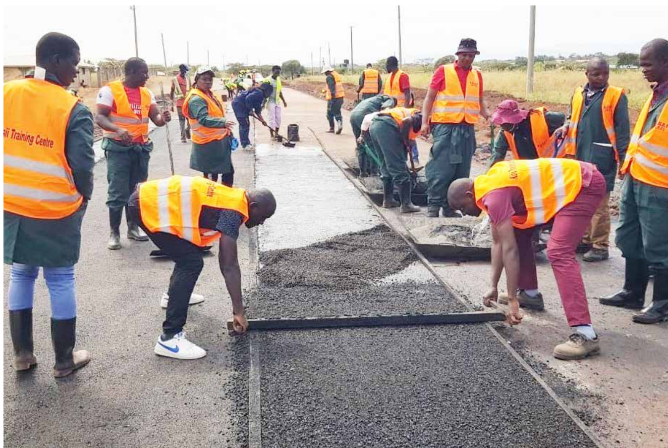
KIHBT Trainers construct roads during industrial attachment.
