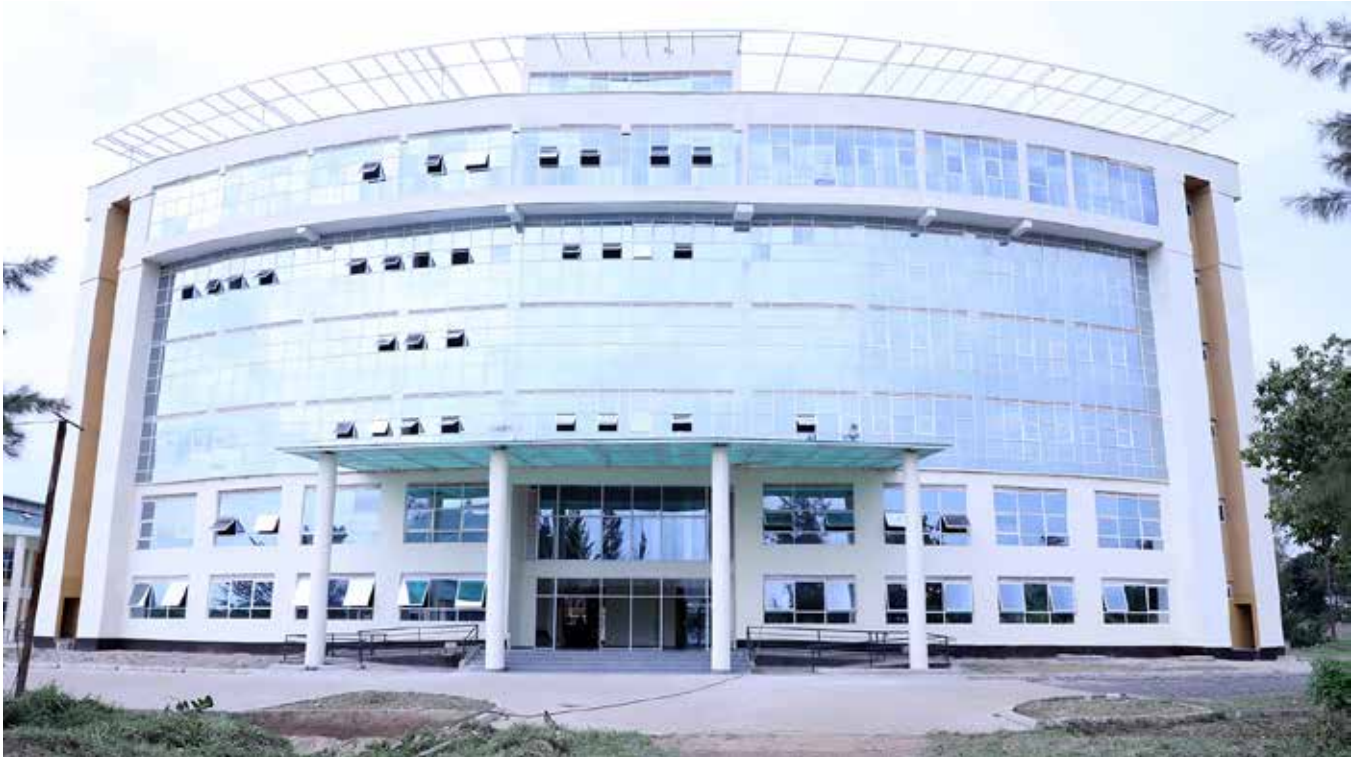
Newly constructed Regional Flagship TVET Institute in Textile Technology at Kisumu National Polytechnic College.
